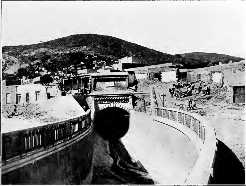
VIEW OF THE PORFIRIO DIAZ TUNNEL, GUANAJUATO.
